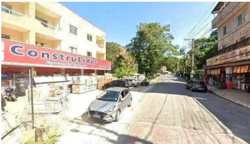
Construlider de mangaratiba street view e 360deg
